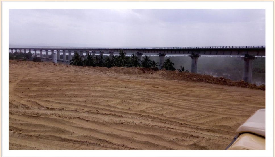
A section of Kenya's Standard Gauge Railway depicting its Engineering Geology magnificence.
